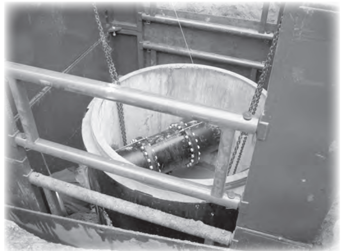
Sewer Manhole Installation - Hemlock Lane
