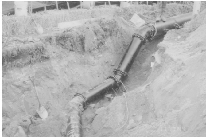
New Water Line Installment Middlesex Turnpike (Photo taken by Dennis Fitzgerald)
